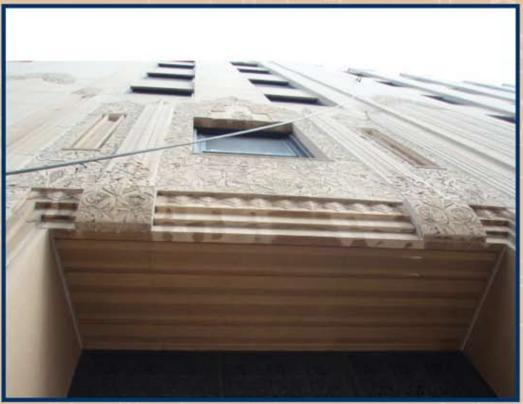
The decorative cast stone panels at the top of the building had undergone severe weathering and deterioration. Their poor condition and fragile state eliminated possibility of removal for creating molds in a controlled environment.
