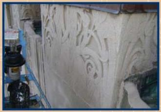
Using swing scaffolds, Corinthian Data Capture's technicians hand scanned the decorative cast stone elements, acquiring a digital map of the intricate surface variations and details.
