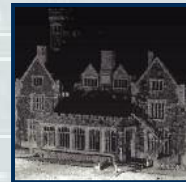
The resulting 3D image can be viewed from any angle, providing a digital database of the building for archive and future reference use in restoration and repair programs.
