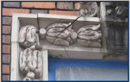
Original broken terracotta – if this was to be removed, it would fall apart resulting in many additional hours of work and significant cost, to put "Humpty Dumpty" back together again.
