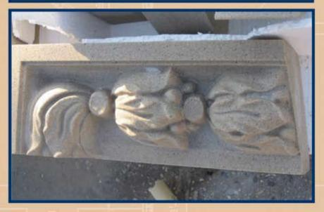
Fabricated cast stone unit to be installed.
